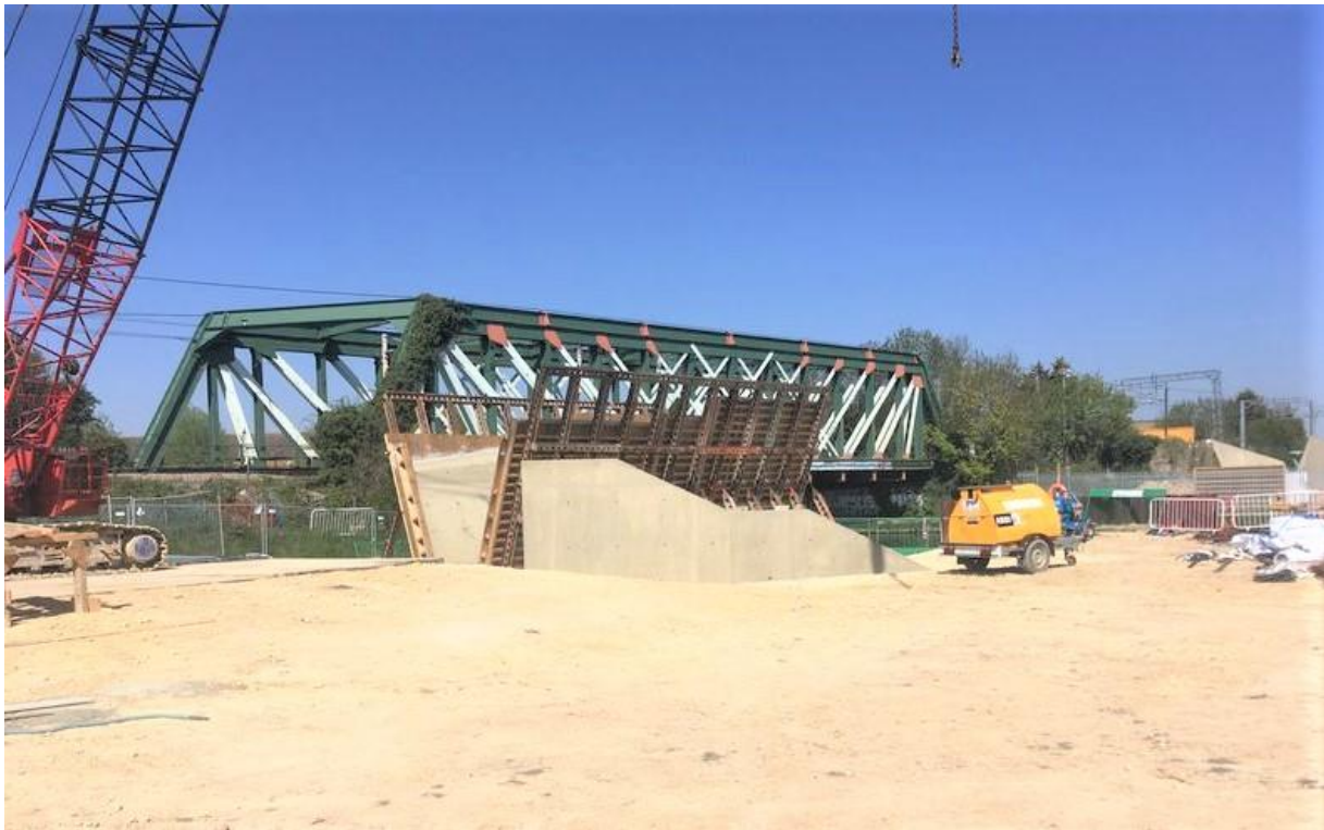
Figure 3. Works in progress on the Chisholm Trail – new bridge for cyclists and pedestrians being installed.
